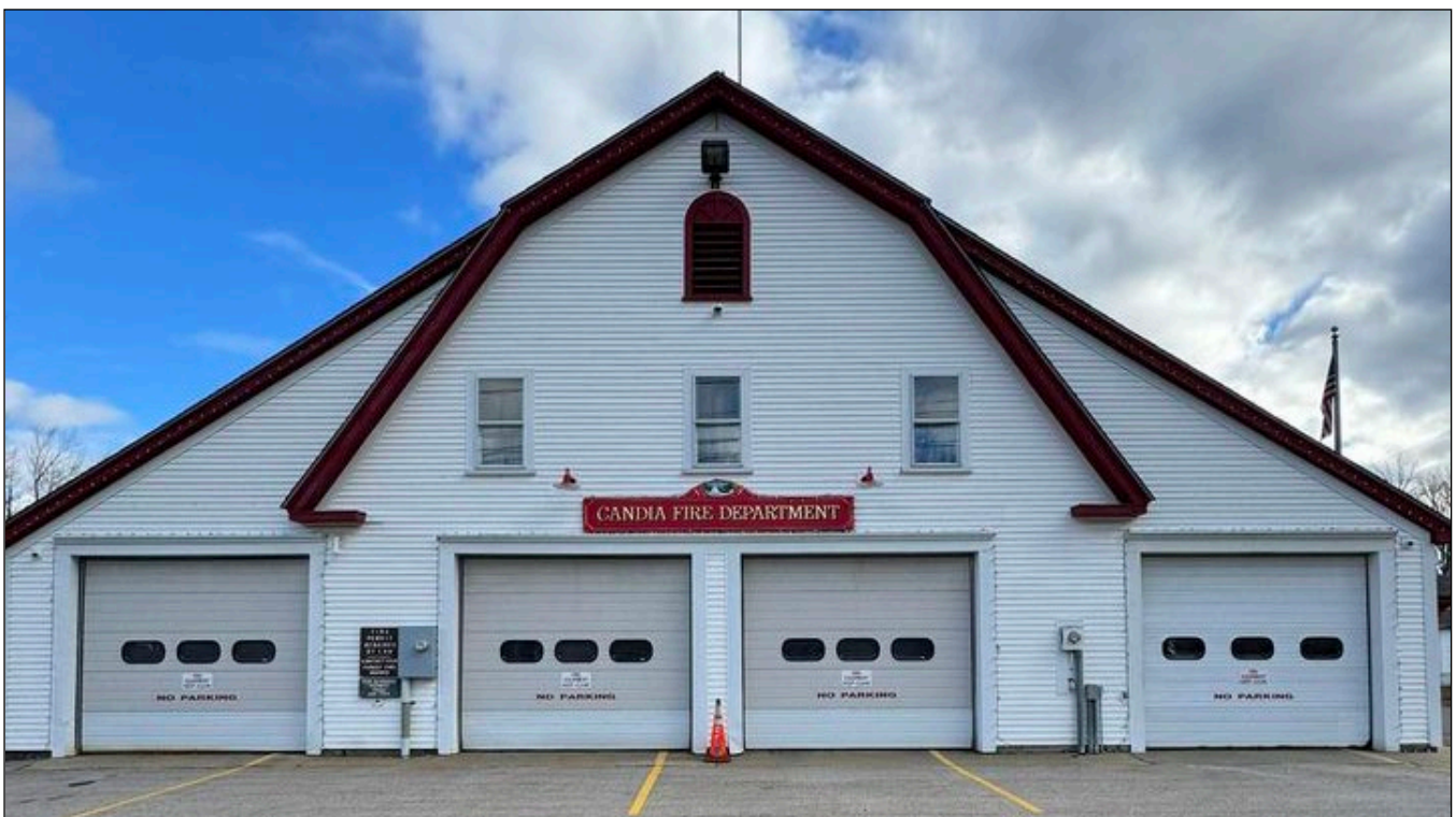
The Candia Fire Station has significant safety deficiencies, including no ventilation system for vehicle exhaust.
