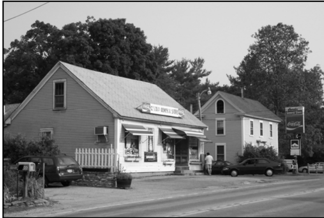
Neighborhood general store located in Candia Village.
